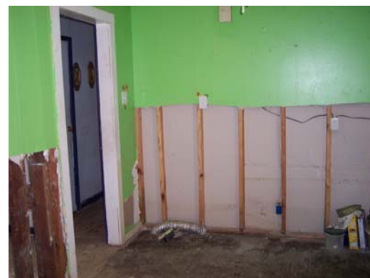
Mold had begun to grow and a church group was able to come in and tear out the wet drywall and insulation. Floors and cabinets will also need to be removed.
